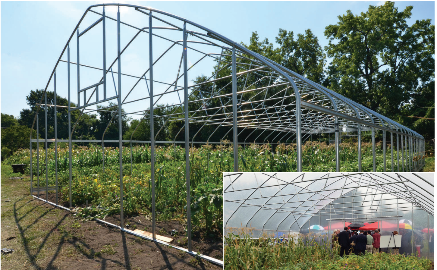
High tunnel installation begins over Avon Standard's vegetable garden.
