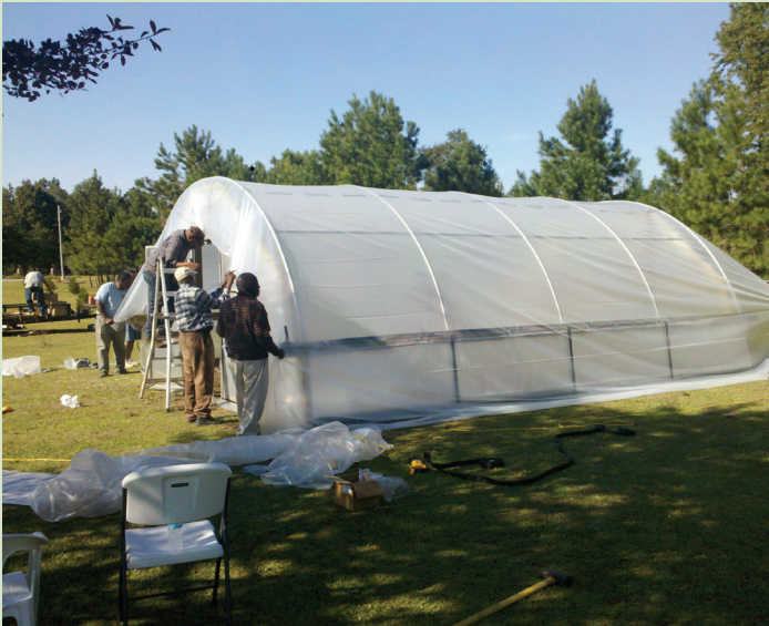
Installation of the plastic covering is almost complete.
