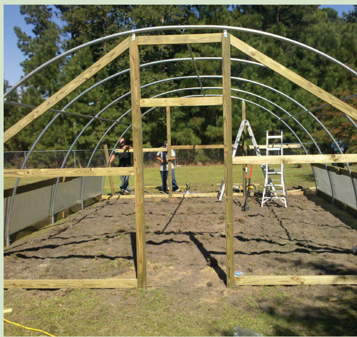
This photo shows wood and metal framing going up.
