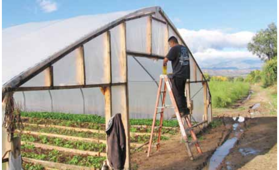
A high tunnel under construction
